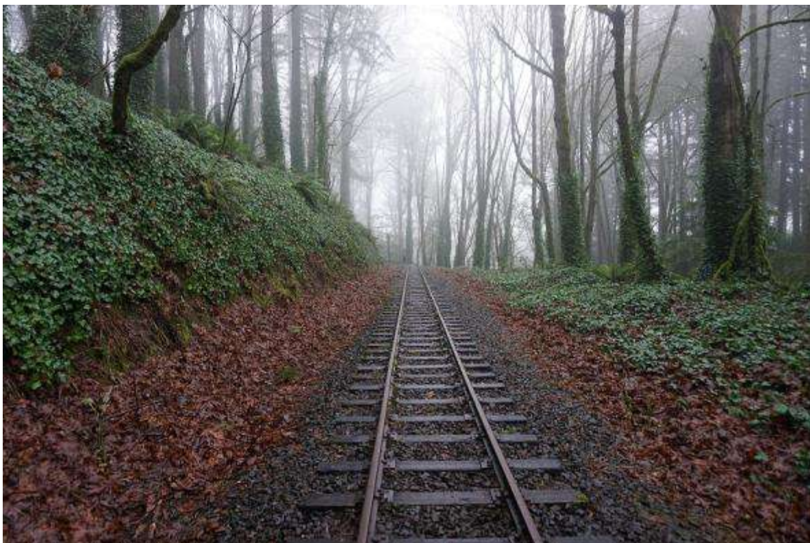
Photo 14 of 21: OR_Multnomah_PortlandZooRailway_0014 Looking north on Washington Park line
