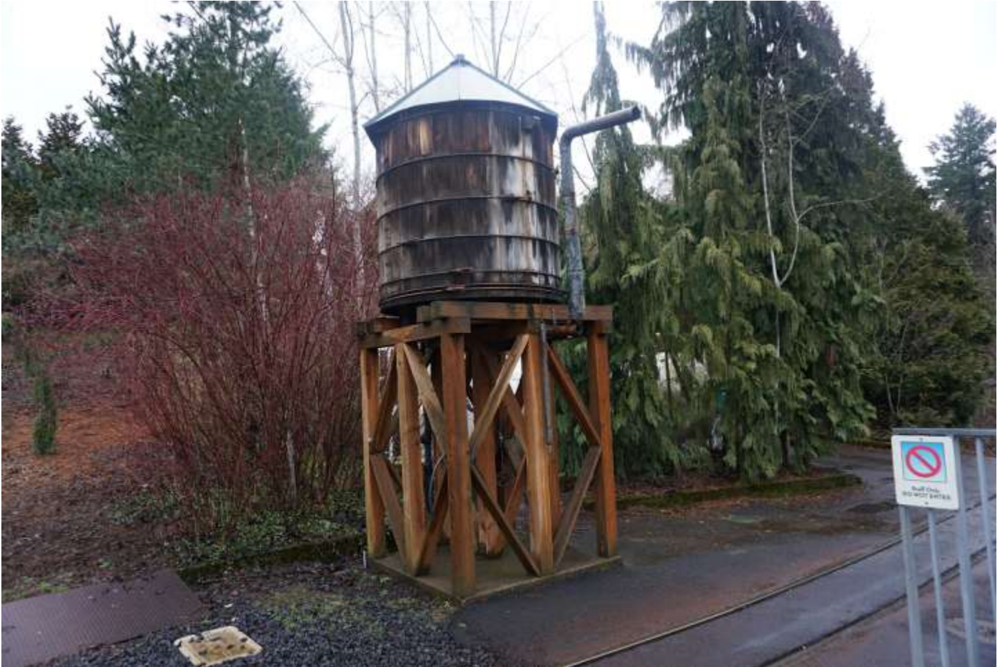
Photo 21 of 21: OR_Multnomah_PortlandZooRailway_0021, water tower looking northeast
