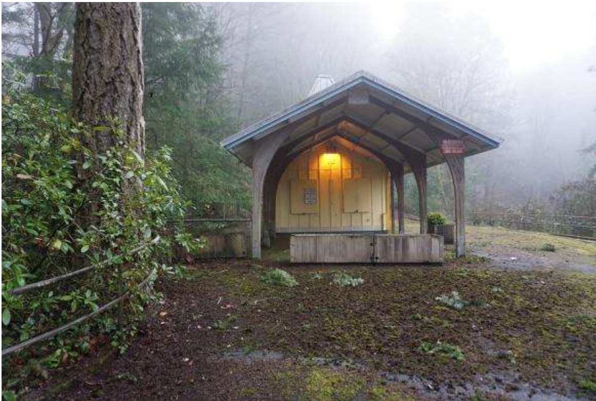
Photo 12 of 21: OR_Multnomah_PortlandZooRailway_0012 East elevation of Washington Park Station looking west
