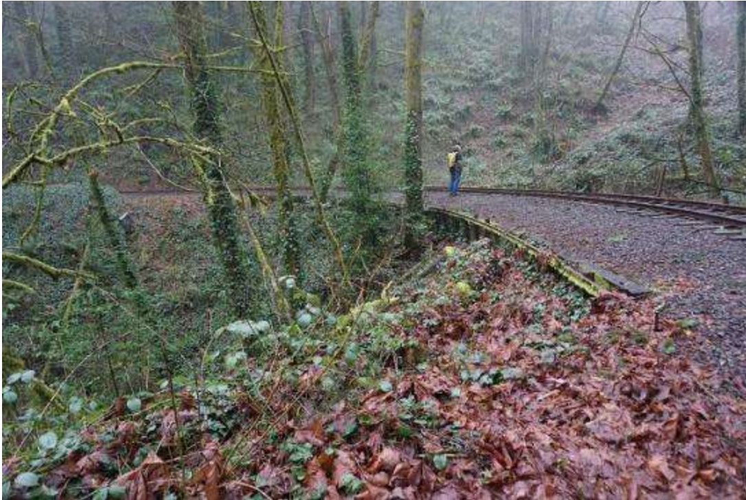
Photo 7 of 21: OR_Multnomah_PortlandZooRailway_0007 Embankment over Texas Gulch, looking southeast
